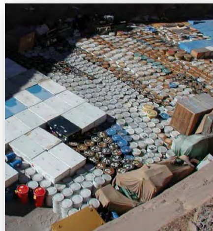
Figure 4: Radioactive and toxic wastes placed for burial in an unlined pit at LANL
